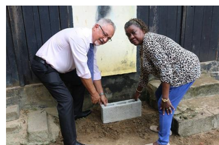
Minister Ferrari and Hon. Regina Esparon laying the foundation stone
